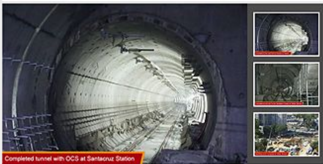
Completed tunnel with OCS at Santacruz Station
