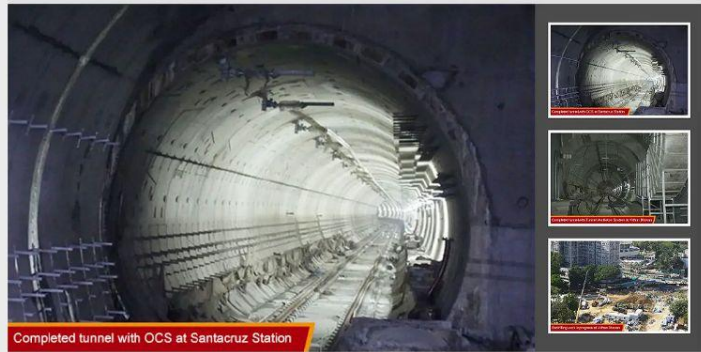
Completed tunnel with OCS at Santacruz Station
